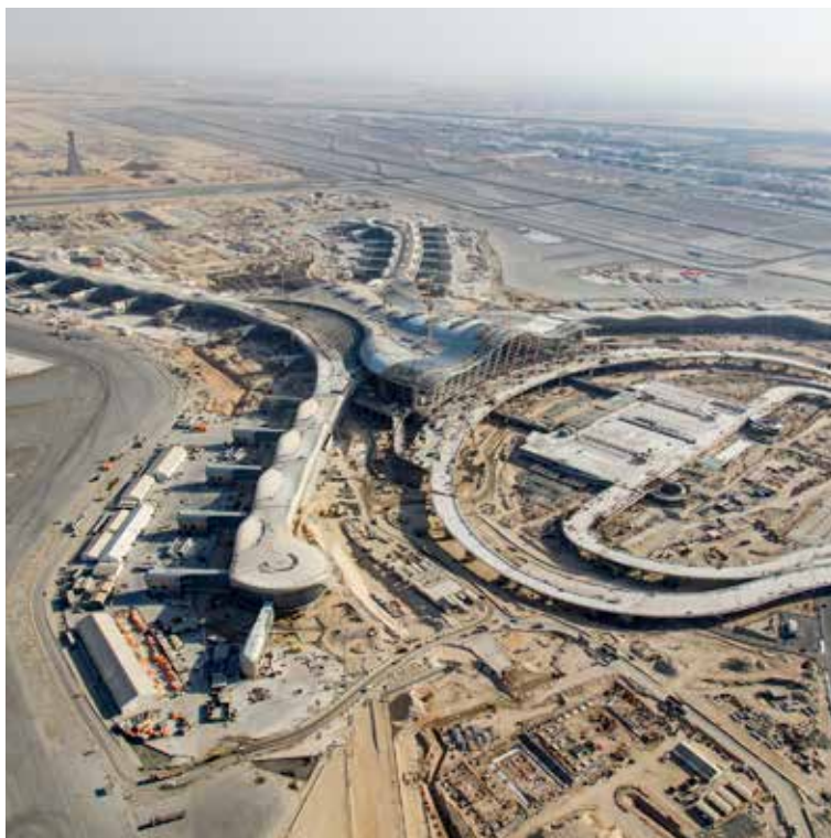
ABU DHABI AIRPORT, ABU DHABI, UAE
